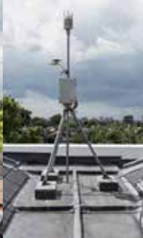
Above: A weather station added by Historic England to monitor external conditions is linked to internal sensors so the performance of the house can be tracked Left: Solar thermal panels, hidden on one of the inner pitches in the roof, supply around half of the hot water used in the house
